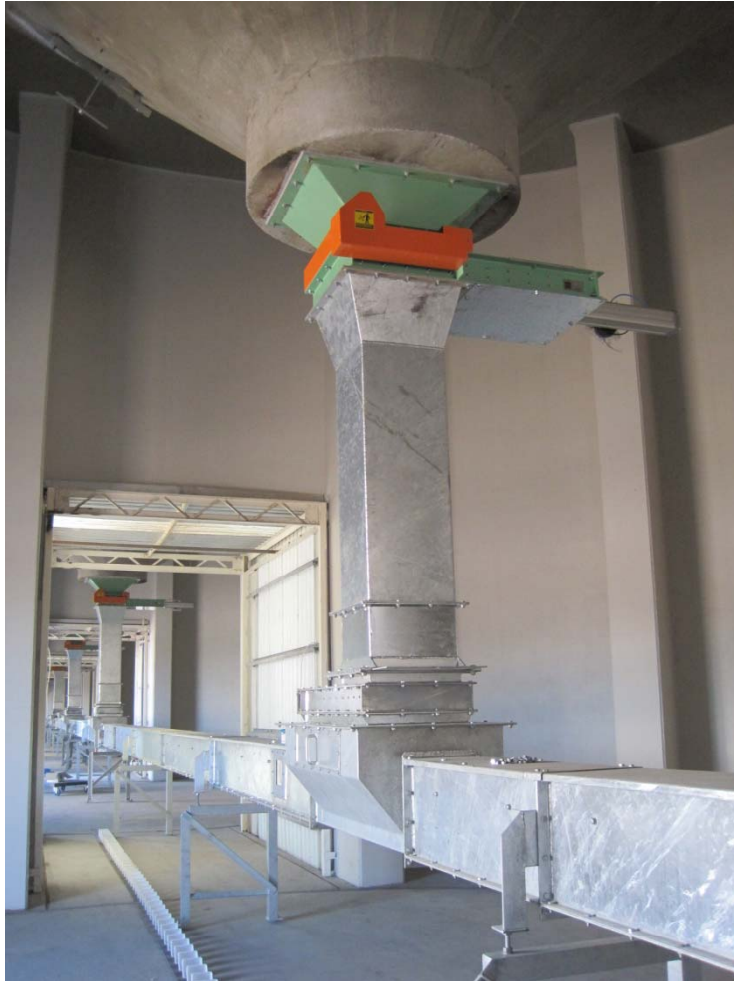
Basement of the Barley Silos
