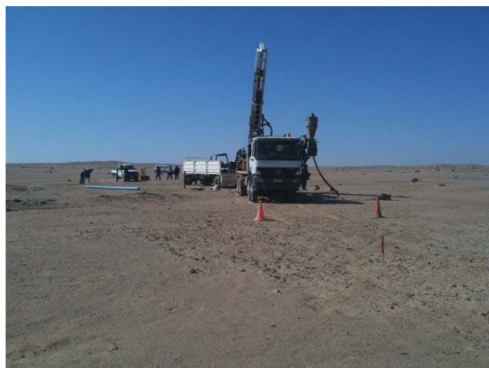
M62 – RC Drilling – June 2010
