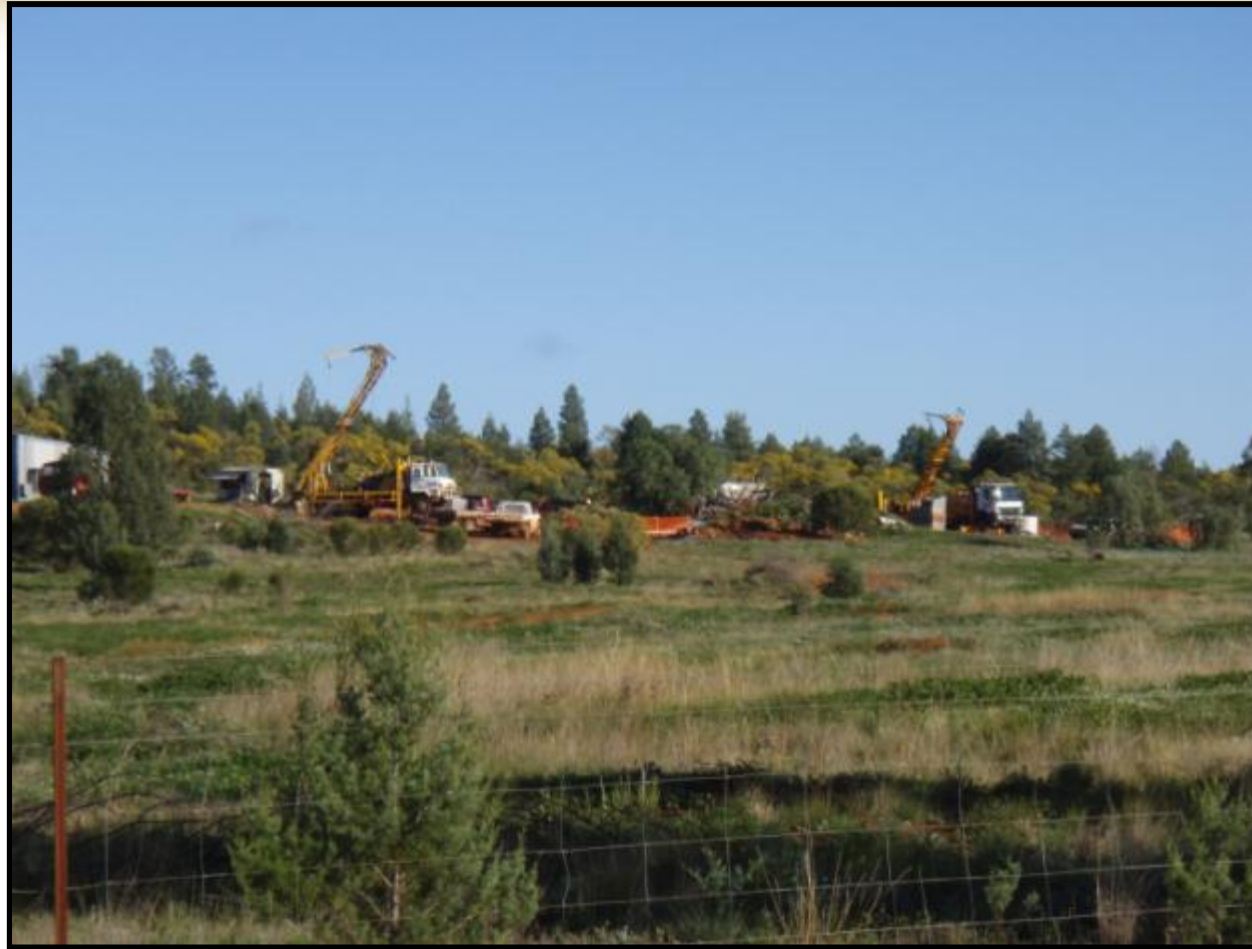
2 Rigs now drilling on Nymagee Copper Mine
