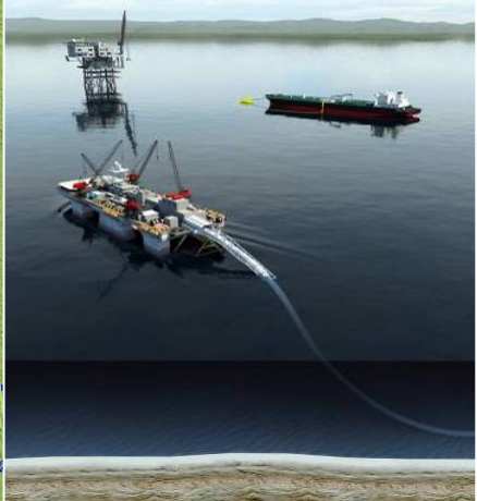
PL 4 (Offshore) ~407km Gas Pipeline
