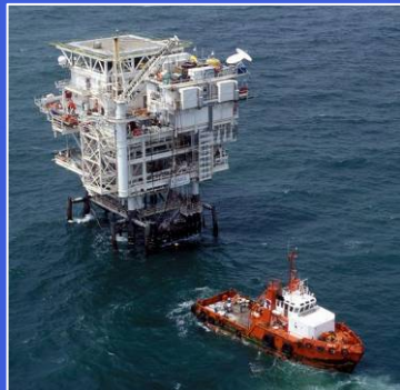
Kumul Marine Terminal
