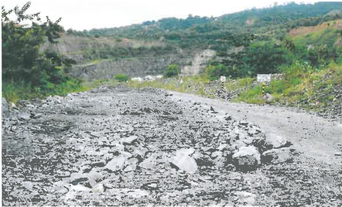
Main Bibiani Open Cut Eastern access ramp being resurfaced
