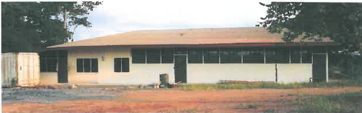
Junior staff refurbished onsite meals facility nearing completion
