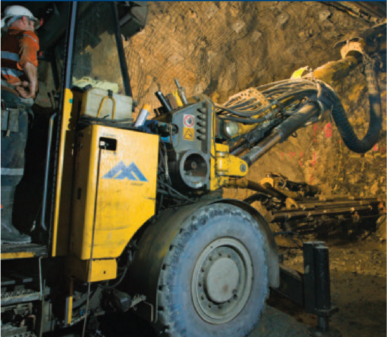
Underground development rig at Renison Mine, Tasmania
