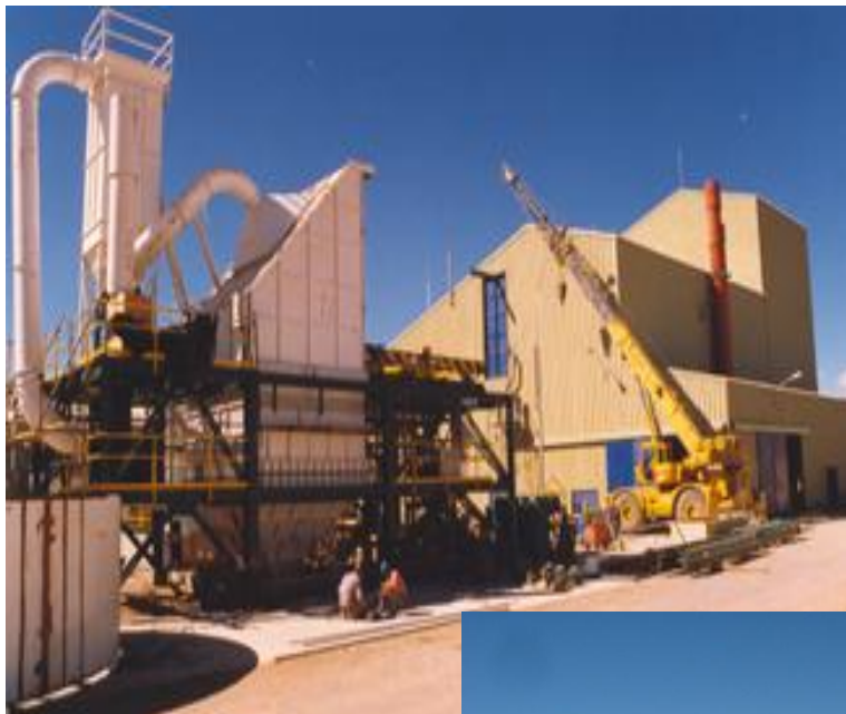
FMC's processing plant at Hombre Muerto
