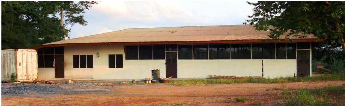
Junior staff refurbished onsite meals facility nearing completion
