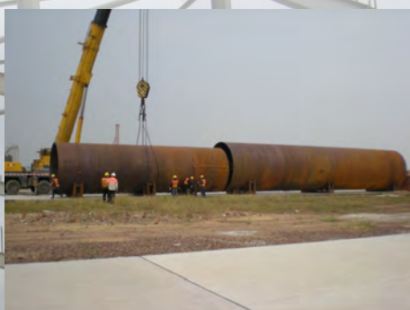
Kiln installed on site
