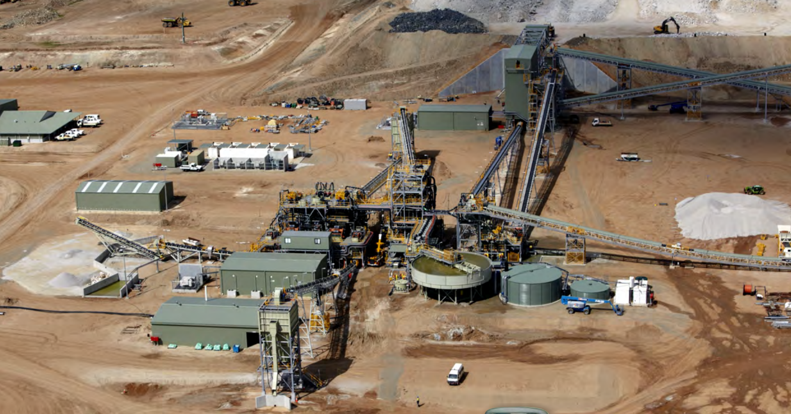
Mt Cattlin Crusher Plant
