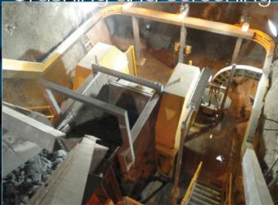
Crushing and screening
