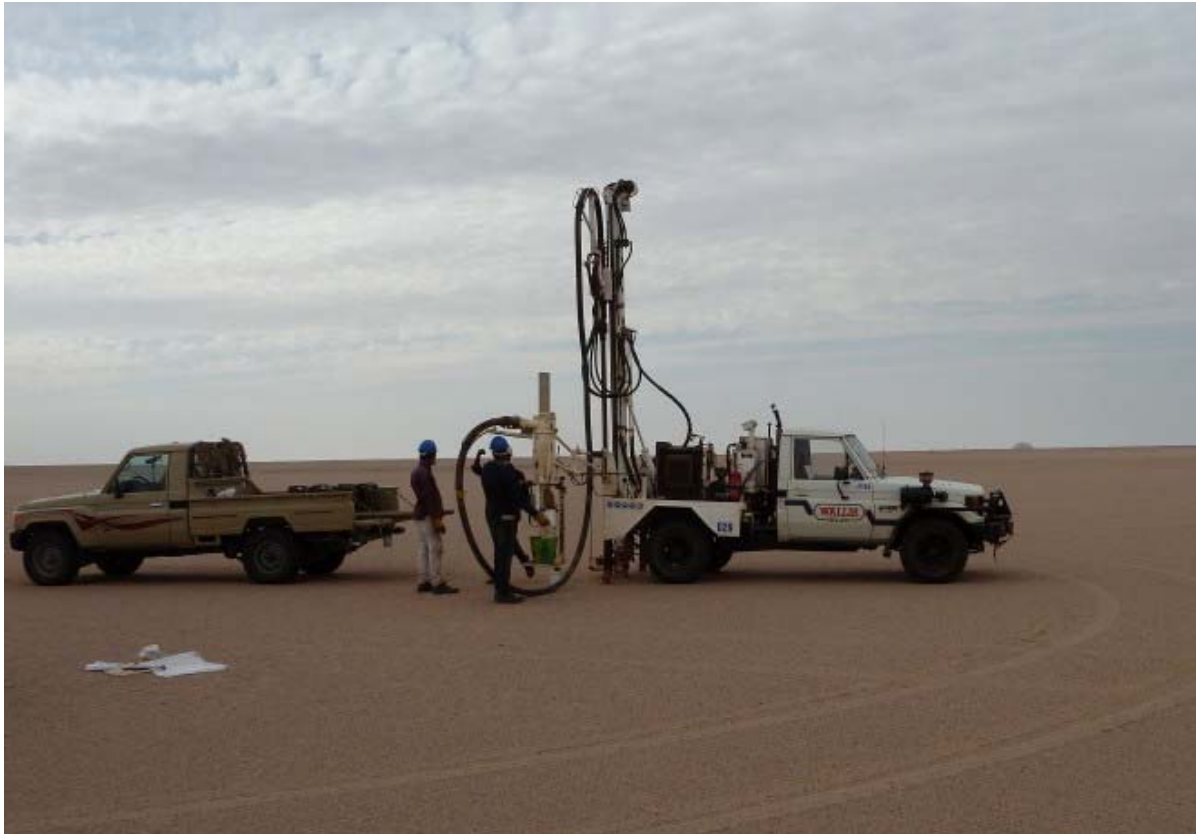
Drill rig on site
