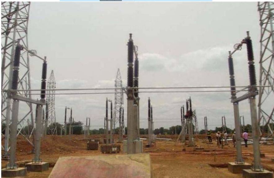
Sikasso Substation Progress July 2010 – 80% completed
