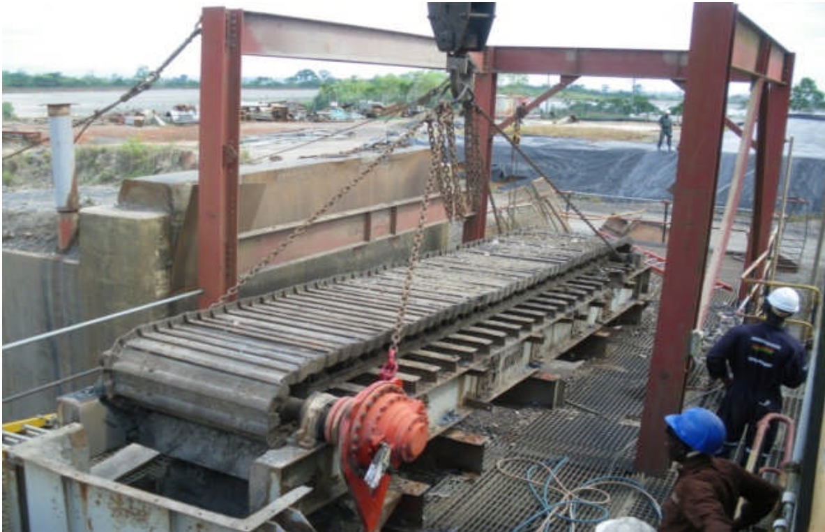
Figure 4 – strip out of the Emergency Feeder Before
