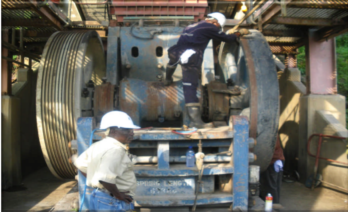
Figure 5 – strip out of the crushing circuit complete
