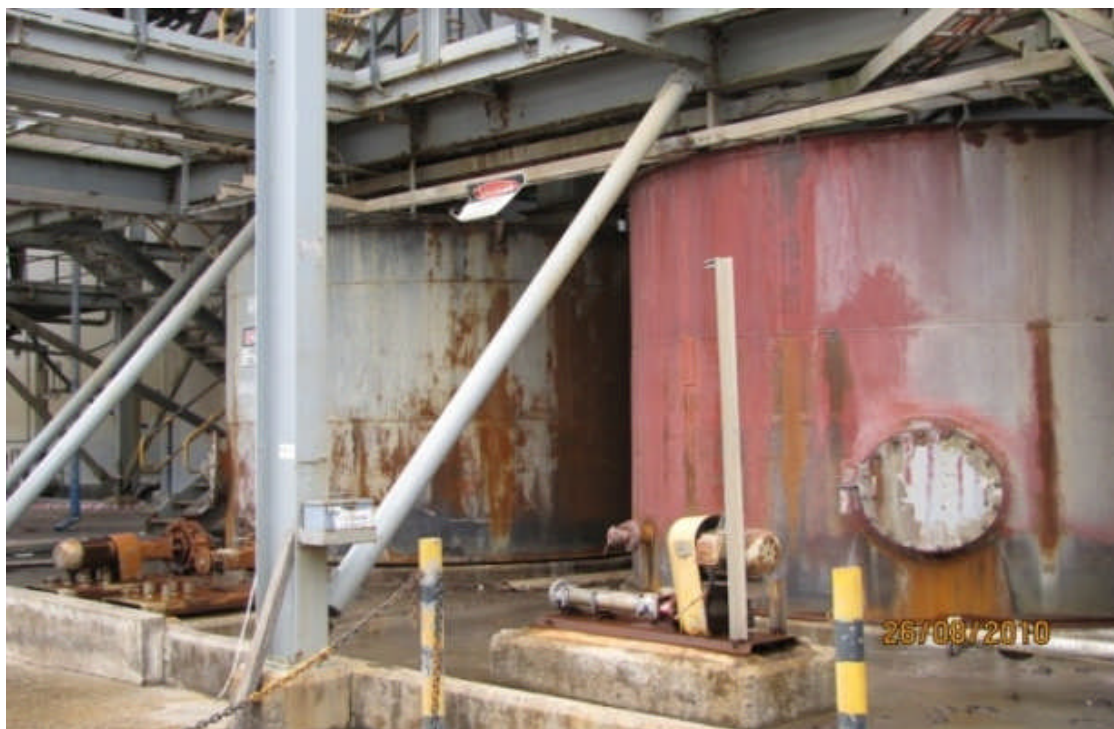
Figure 6 – strip out of the cyanide mixing tank complete
