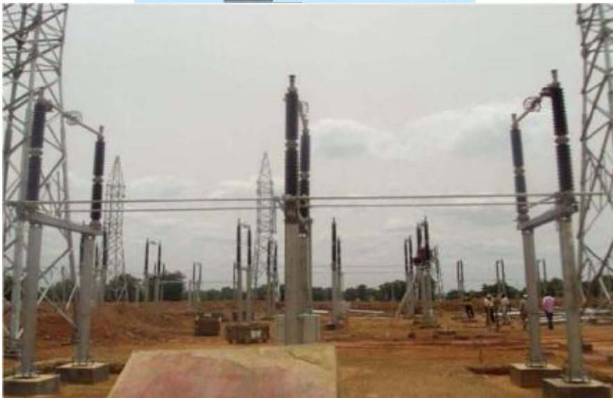
Sikasso Substation Progress July 2010 – 80% completed
