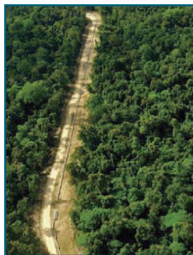
Pipeline stringing, onshore pipeline
