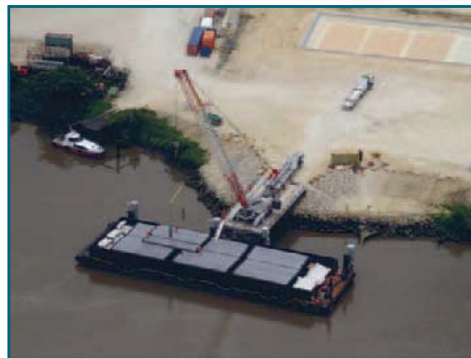
Pipe offloading at Kopi Shore Base
