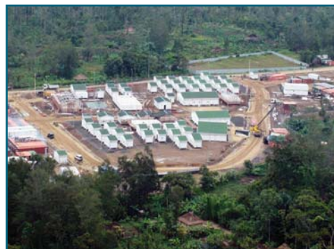
Komo Camp construction
