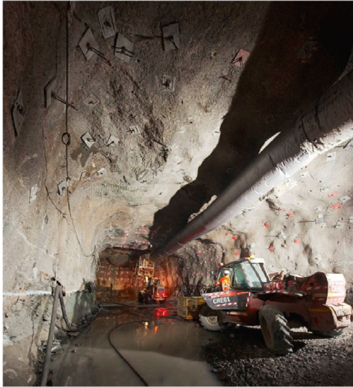
Argyle diamond mine, Western Australia
