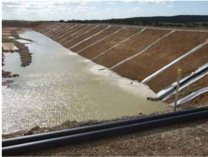
Figure 8.11 Inside of TSF, looking towards north-west corner.
