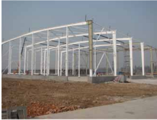
Figure 9.5 Steel Structure of Lithium Product Warehouse and Lithium Packaging Building
