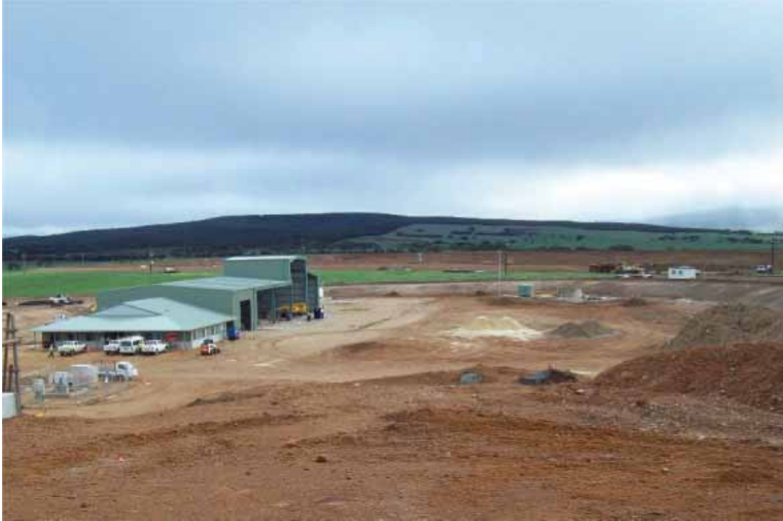
Figure 8.9 Workshop Building with Tailings Storage Facility in Background.
