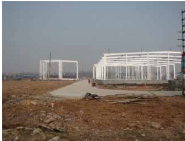
Figure 9.5 Steel Structure of Lithium Product Warehouse and Lithium Packaging Building
