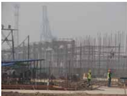
Figure 9.8 View of some of the conveyer work from the port
