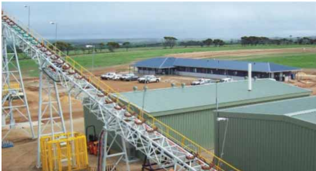
Figure 8.8 View over Laboratory to Administration Building
