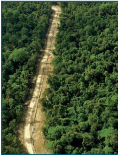
Pipeline stringing, onshore pipeline
