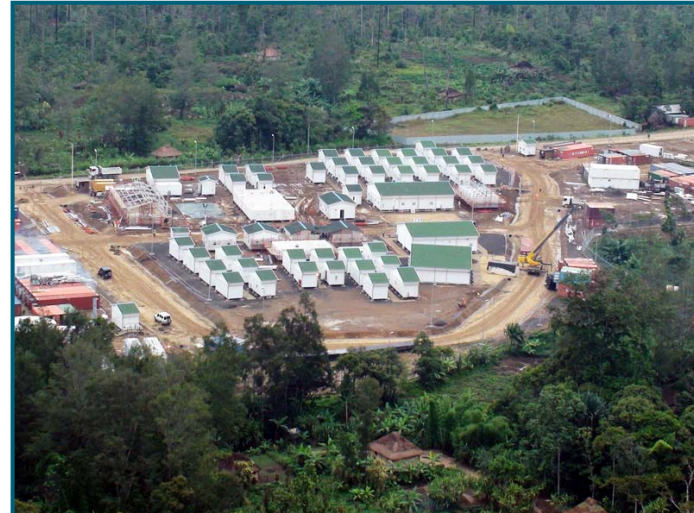
Komo Camp construction
