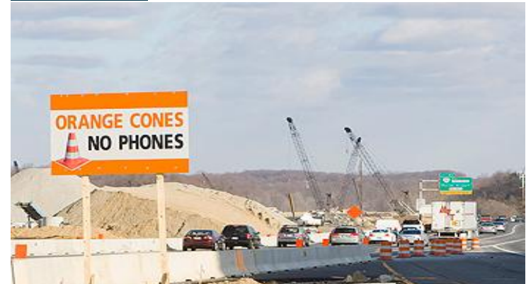
On-road signage reaches Beltway drivers in the construction zone.
