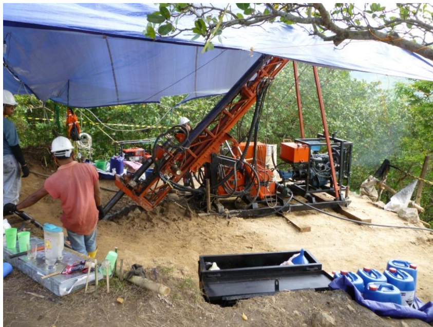
Drilling at Randu Kuning
