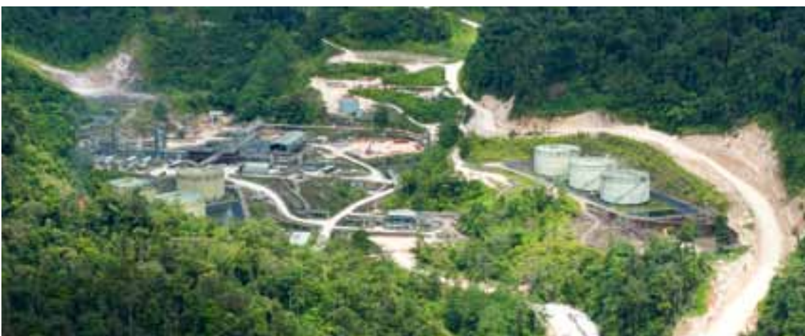
Left: Central Processing Facility (CPF), Kutubu
