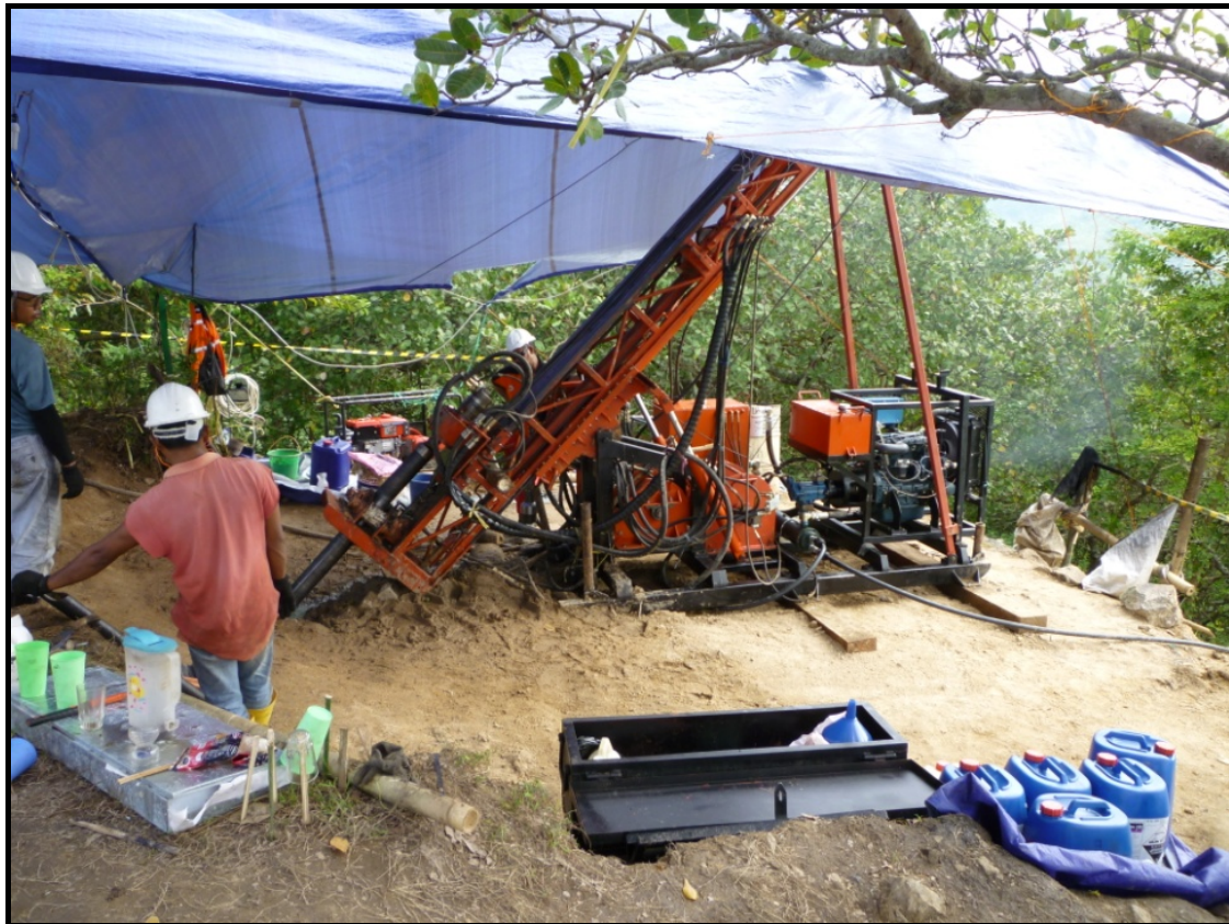
Drilling at Randu Kuning
