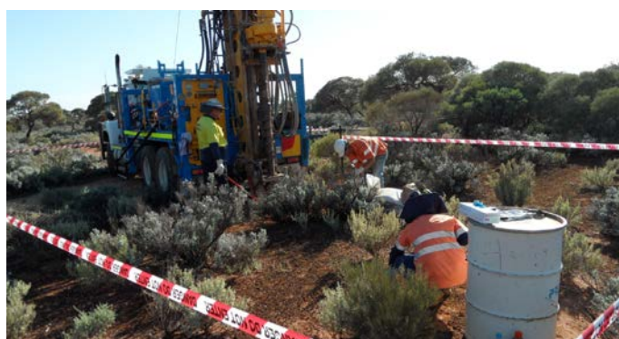
Groundwater monitoring bore being installed by Drilling Solutions, and soil sampling being conducted by AECOM, as part of the Whyalla site EIS program (March 2011).
