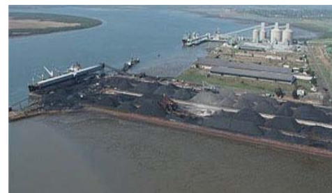
Matola coal terminal, Maputo
