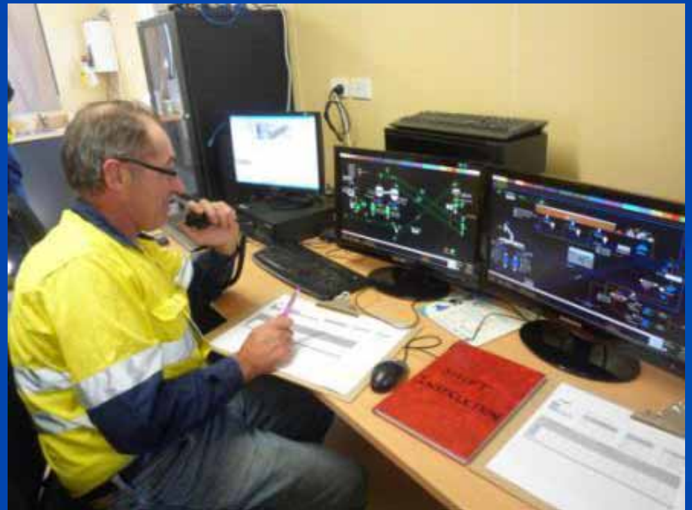
Mt Cattlin control room
