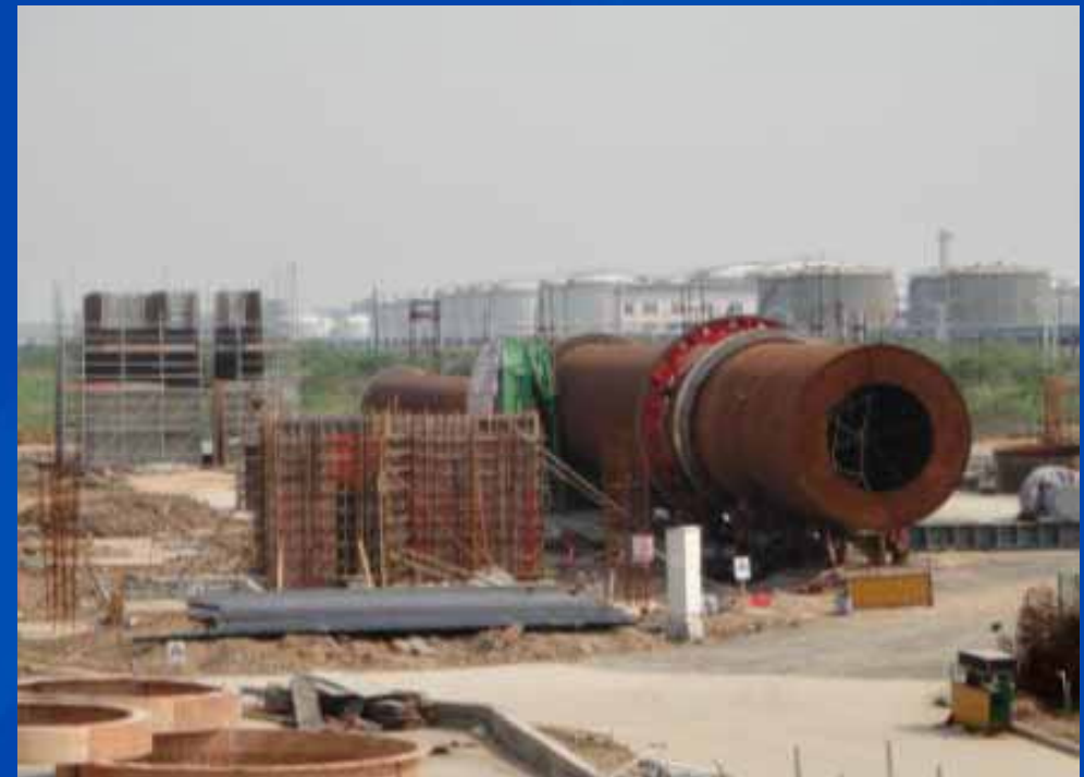
Calciner construction on site
