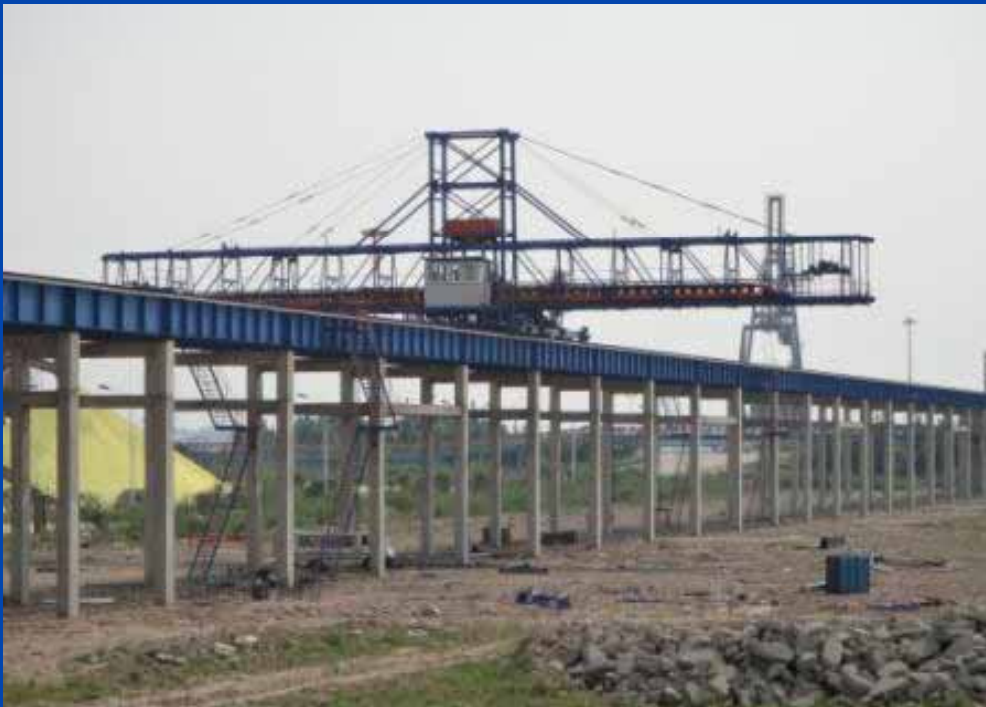
Conveyor construction to wharf
