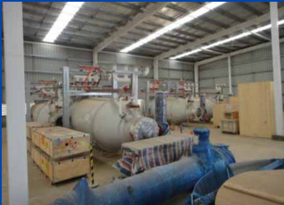
Major equipment on site
