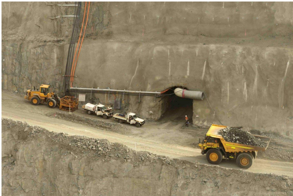
Spotted Quoll underground mine decline portal
