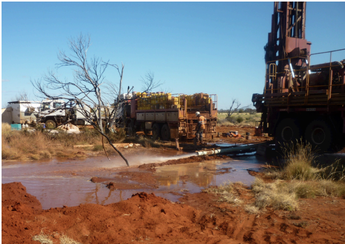
Water flow from water exploration drilling for the Wingellina Nickel Project
