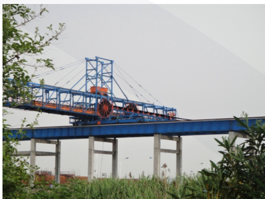
Conveyor from Wharf - Jiangsu, China
