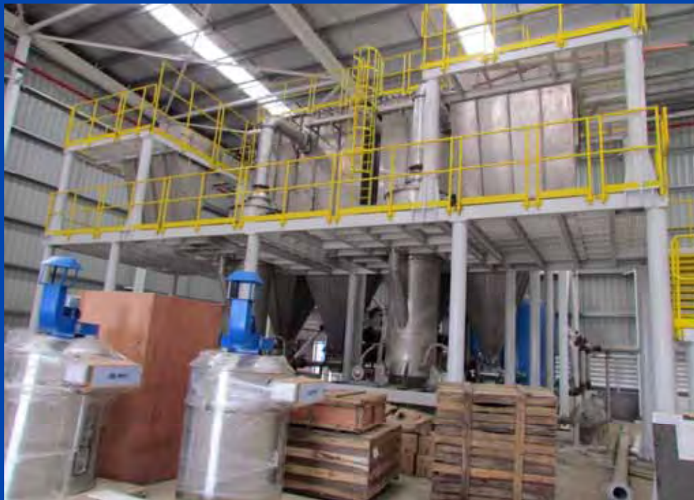
Major equipment on site
