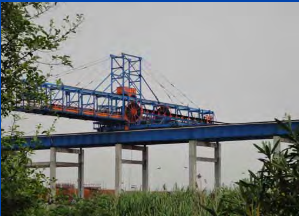
Conveyor construction to wharf
