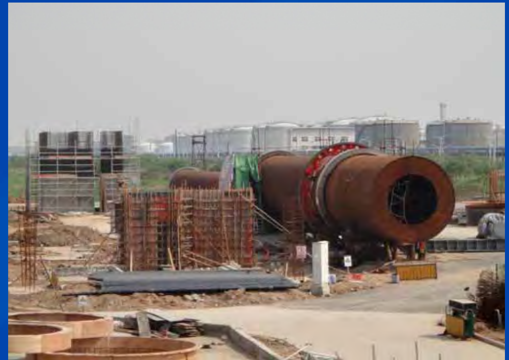
Calciner construction on site
