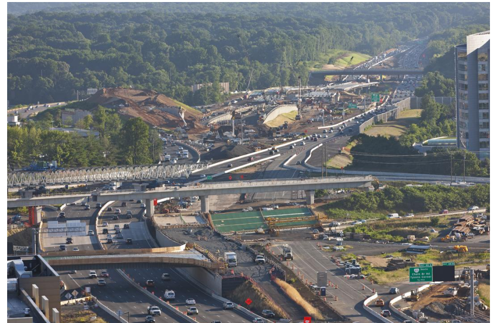
CHAIN BRIDGE ROAD INTERCHANGE
