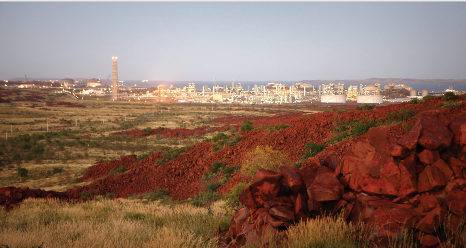
The Woodside operated North West Shelf Karratha Gas Plant
