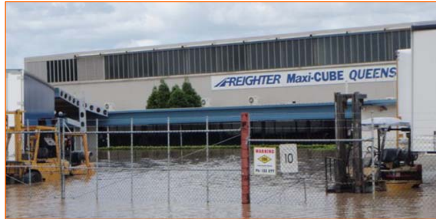
FMQ Head Office flooded Jan. 2011
