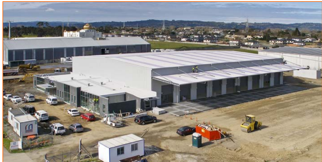
New Auckland Facility nearing completion
