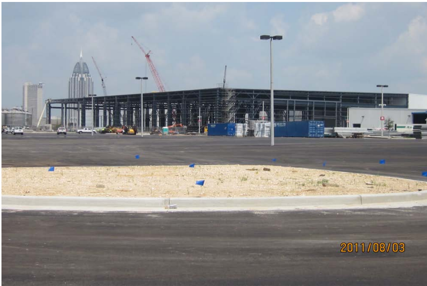
Modular Manufacturing Facility
