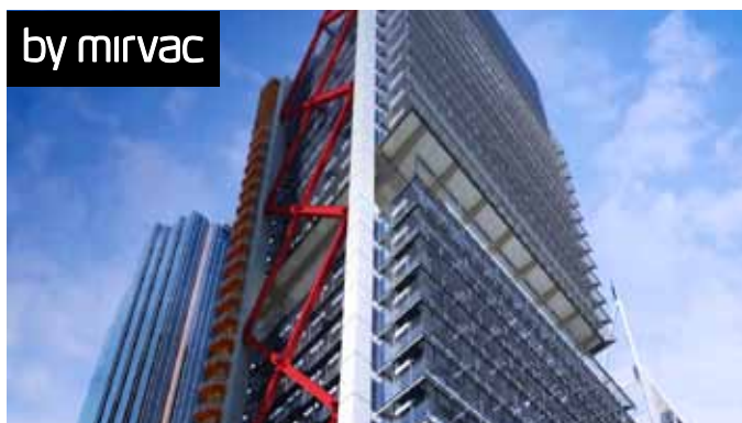
8 CHIFLEY SQUARE, SYDNEY, NSW IN PROGRESS
