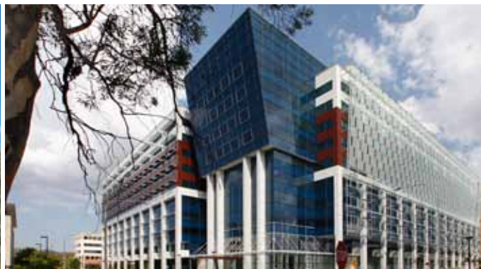
SIRIUS BUILDING 23 FURZER STREET, PHILIP, ACT
