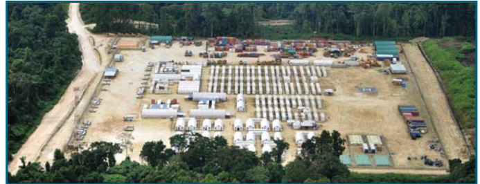
Kopi Scraper Station
