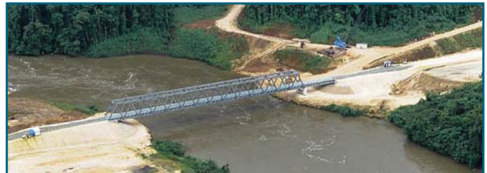
Completed Mubi River crossing
