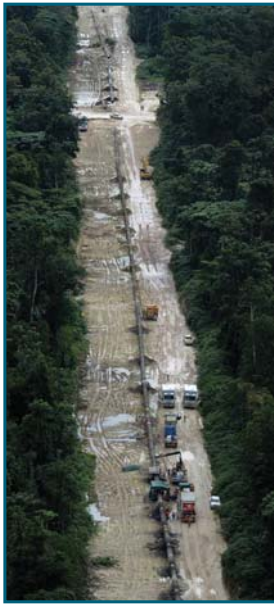
Pipeline stringing, onshore pipeline
