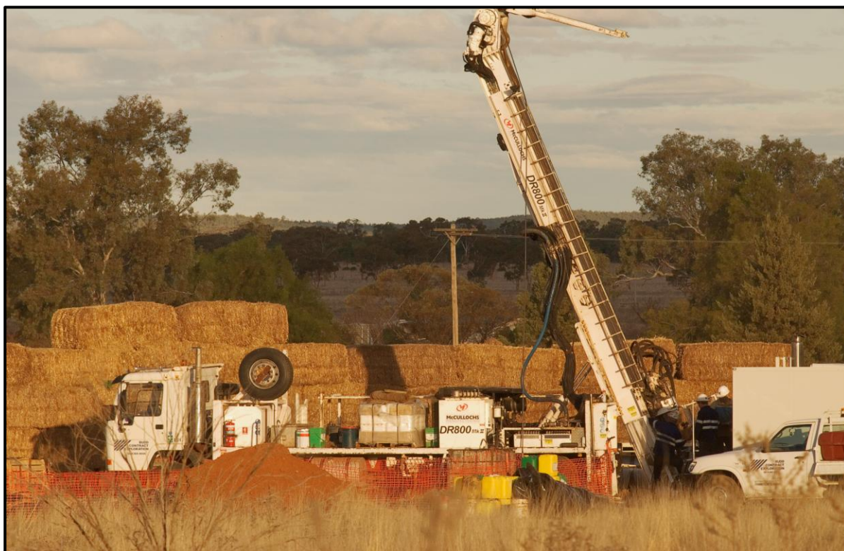
Deep drilling underway – Nymagee Copper Mine
