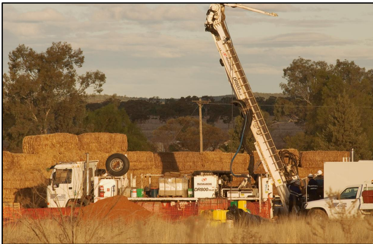
Deep drilling underway – Nymagee Copper Mine
