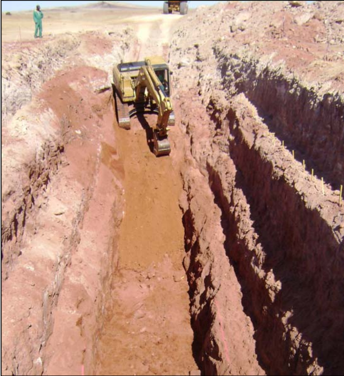
Figure 7: TRS Bulk Sample Trench
