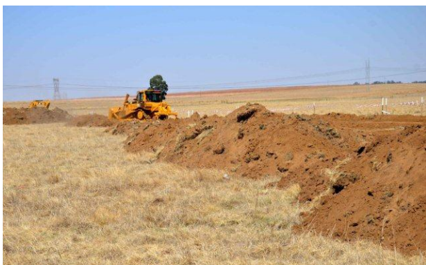
Top soil removal of the box-cut area
