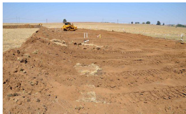
Top soil removal of the box-cut area
