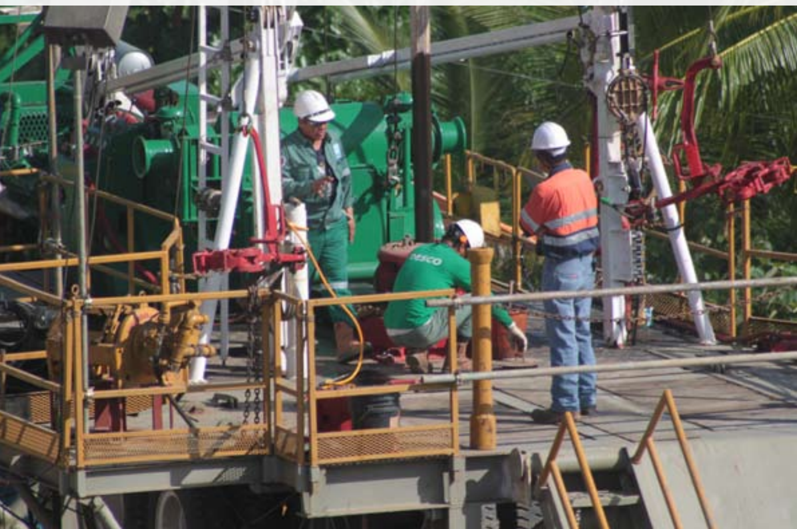
Duhat-1 Rig Crew Checking Equipment
