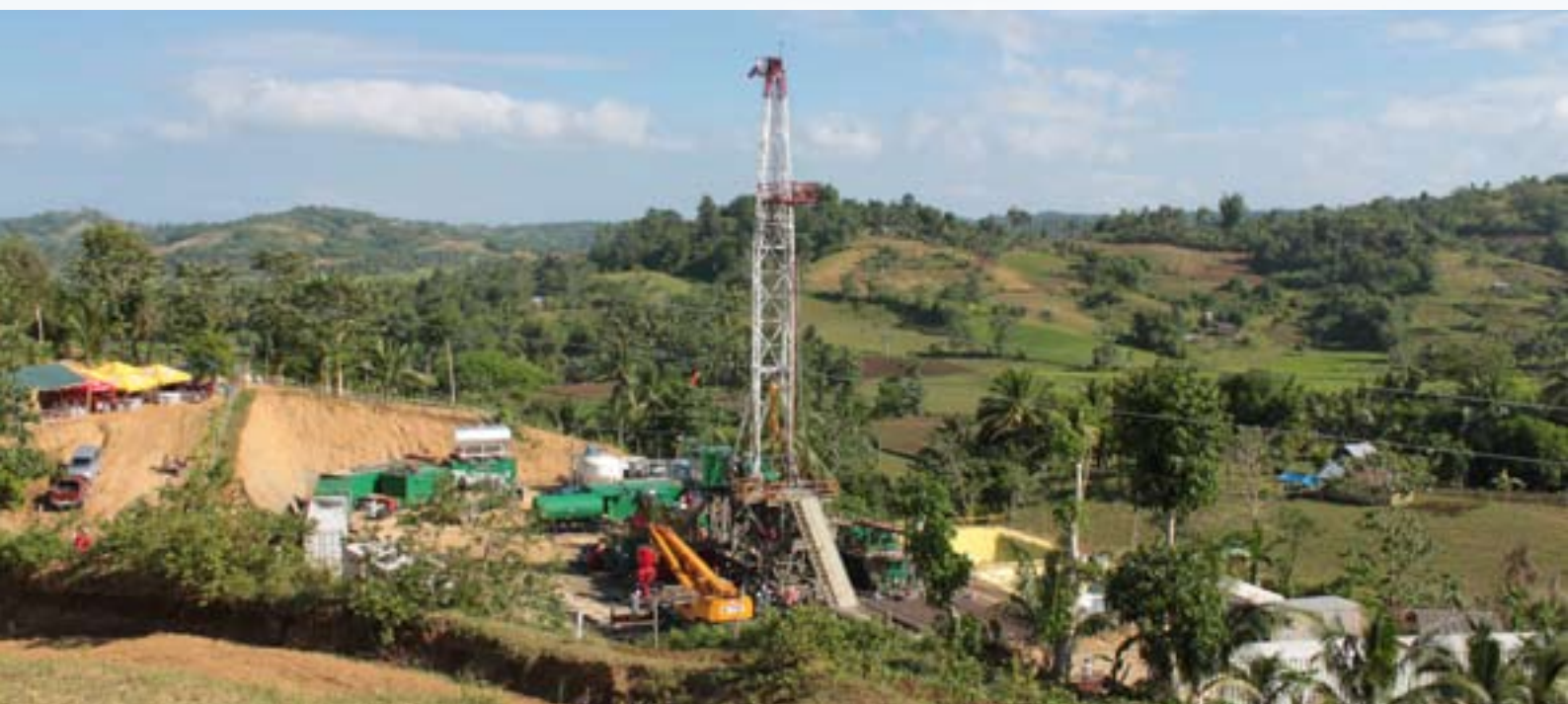
Duhat-1 Rig setup nearing completion
