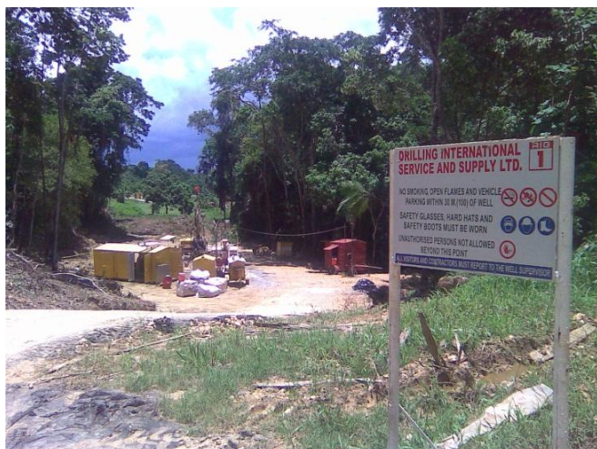
Figure 4 – Rig 1 on Location in Trinidad
