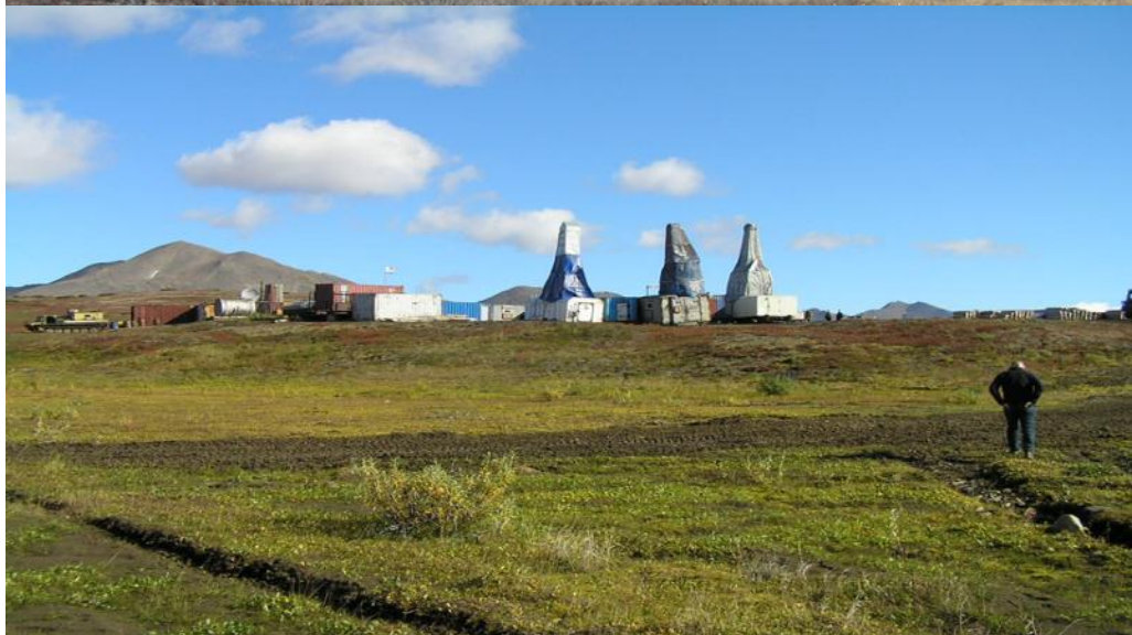
Amaam field camp under construction
