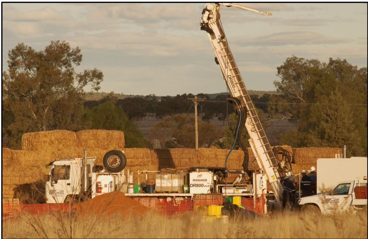
Deep drilling underway – Nymagee Copper Mine
