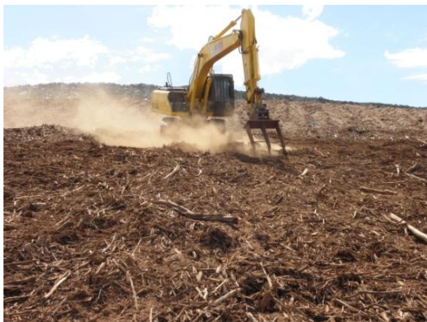
Placing habitat logs on waste dump
