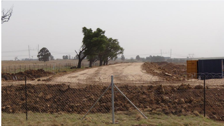
Security fencing and berms have been completed around the project site
