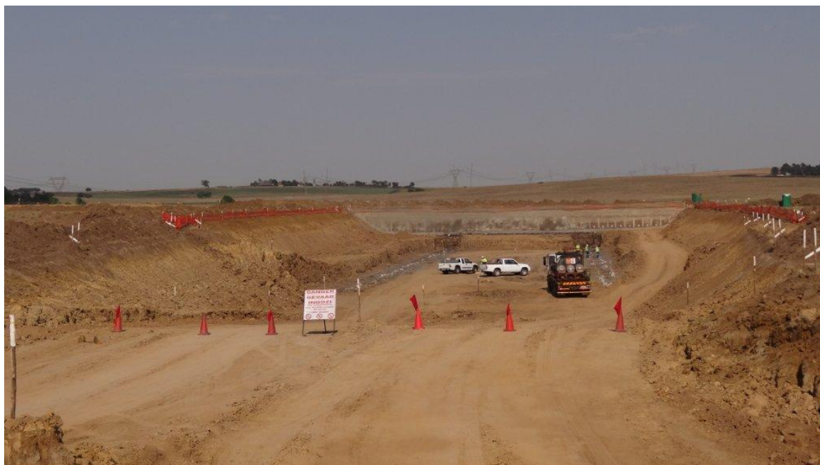
Development activities progressing in box-cut at the Penumbra Coal Mine
