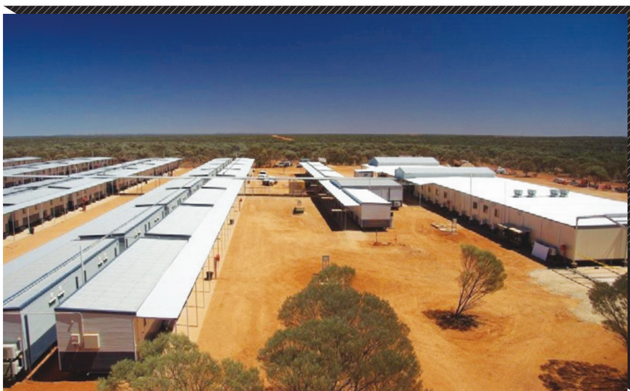
Construction of 250 man camp is nearing completion
