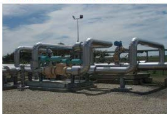
Station reversal skid, Springhurst
