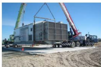
Installing the compressor station at Marsden
