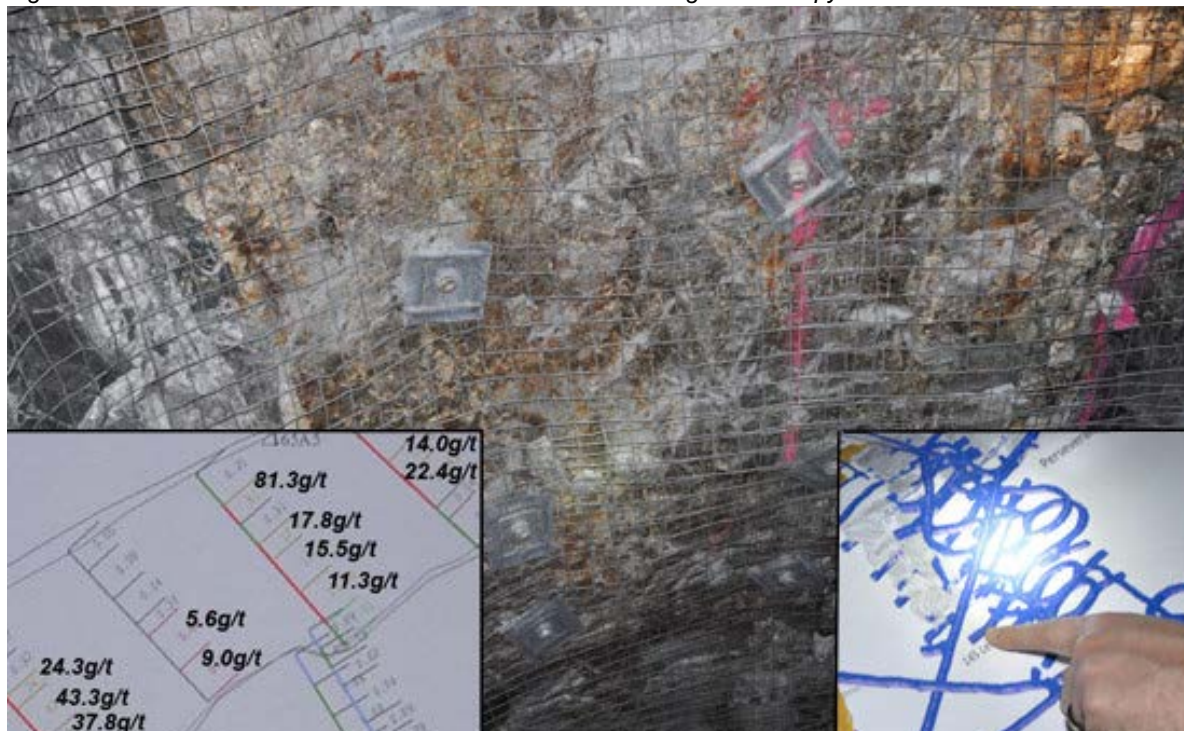
Figure 1: Perseverance Level 145 Main Lode roof South showing extensive pyrrhotite mineralisation
