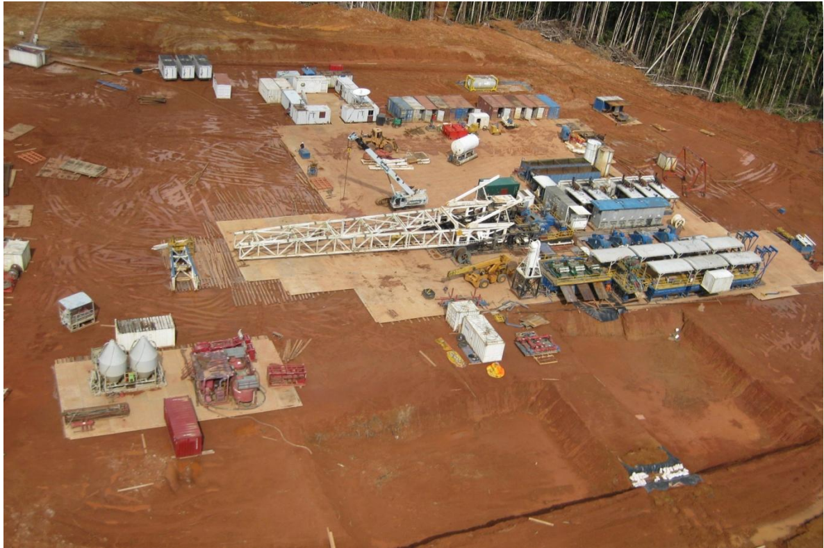
Aerial view of Elevala-2 well location
