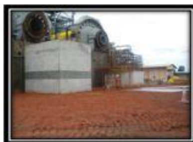
Mill Discharge Pump Civil Works
